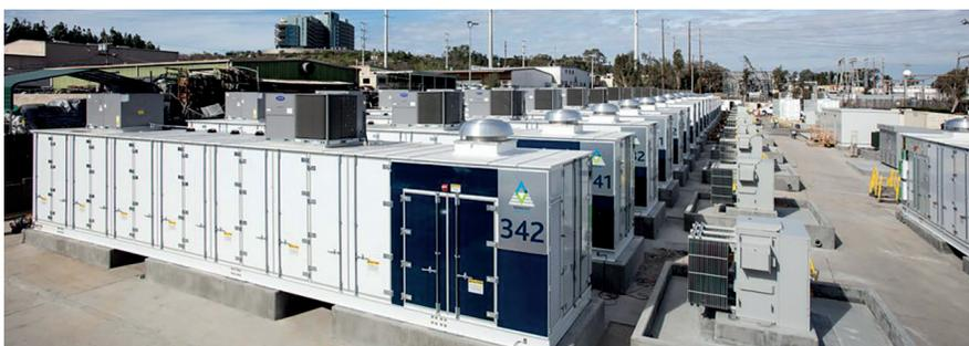
30 megawatt storage system that offer a 4 hour duration for San Diego Gas & Electric in Escondido, California. Source: Fluence.
